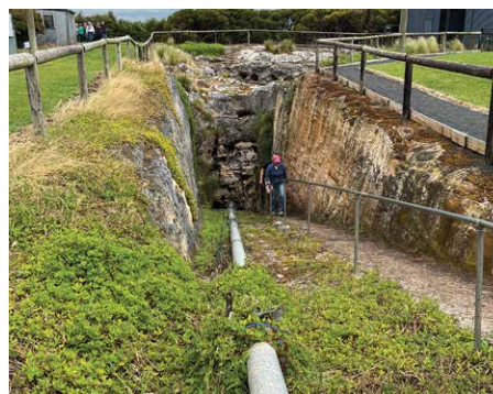
Kilsby Sinkhole Access
